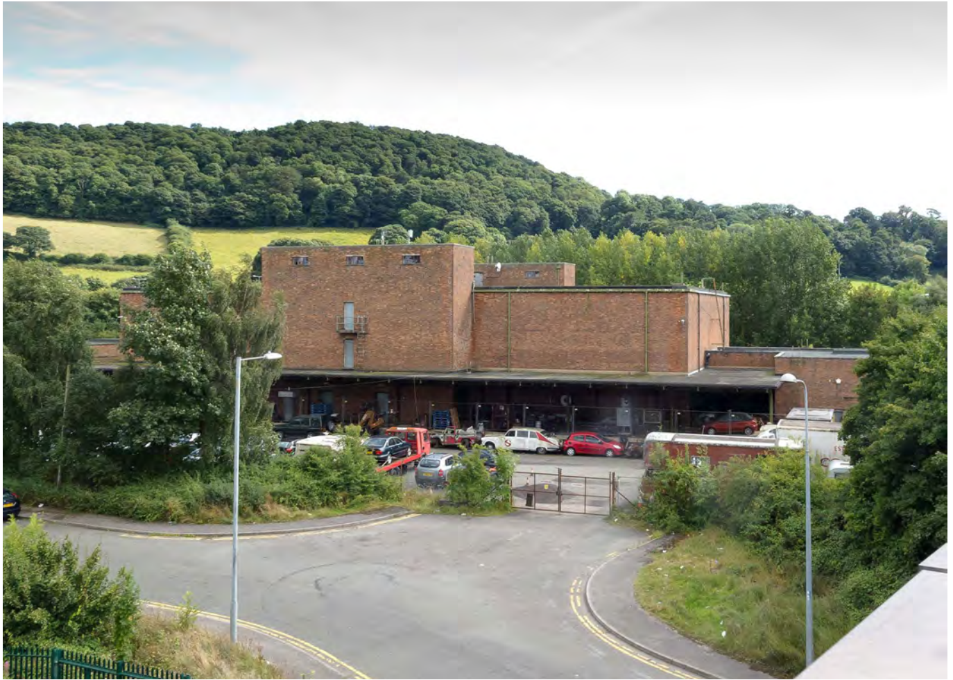
The Marl Cold Store at Llandudno Junction in 2016. Photo Russell Barnes
